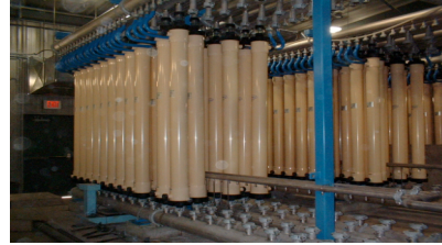
Microfiltration water plant, Petrolia, PA
